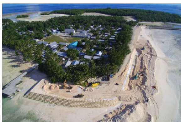
Figure 9-13: Borrow pit filling project at Funafuti (Source: [35])
